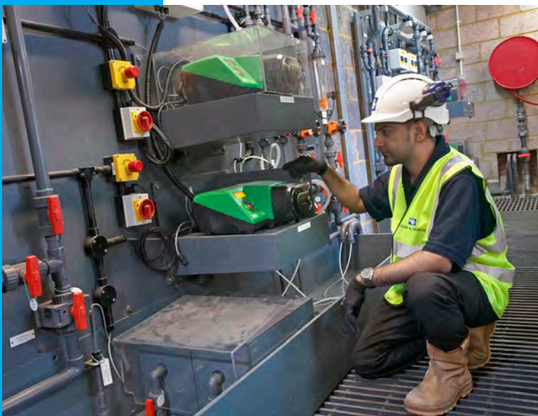
Peristaltic is delivering reduced maintenance on chemical dosing rigs at Severn Trent Water.
