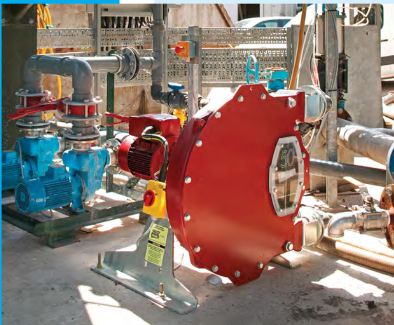
Greencore Group Plc achieved significant savings in downtime and repair costs on the water treatment plant at its Greencore Grocery site thanks to a Bredel 50 high pressure hose pump.
